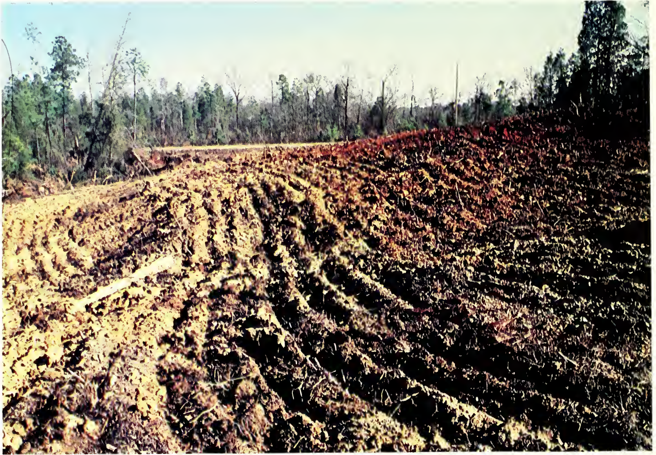
Figure 11.—Mechanical site preparation by disking.
